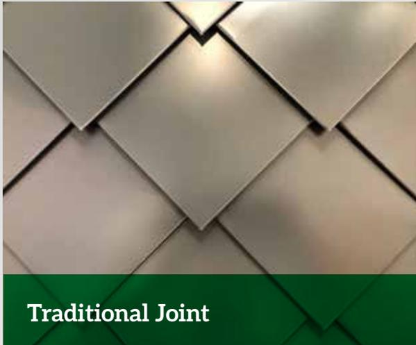
**Description:** A traditional flatlock welded joint with 25mm returned edges interlocking into one another
